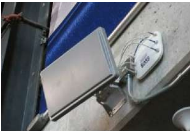
Fig 4. Cisco 3502P AP with Grayling Antenna
